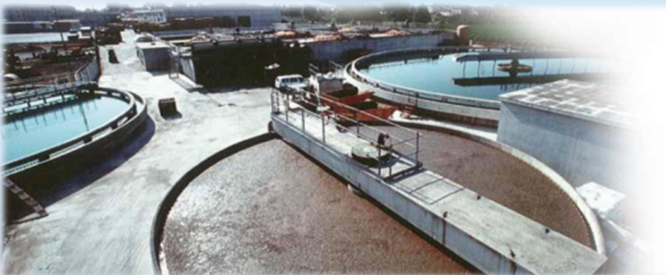
Plant view of food water treatment plant.
