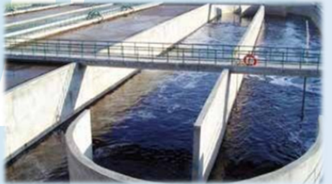
Oxidation tank carousel type - Q = 10.000 m 3 /day.
